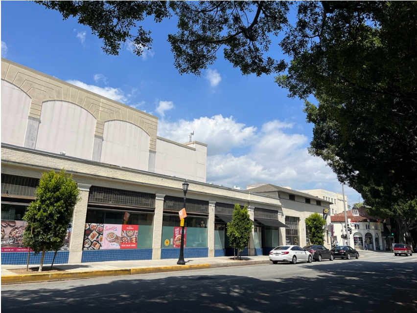
PASADENA: Ficus trees planted in Pasadena in March 2023 to fill in bare spaces in the canopy (picture taken April 27, 2024).
