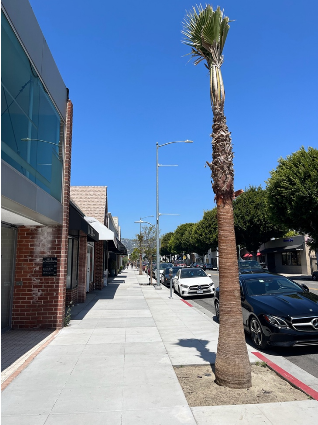
BEVERLY HILLS: View of new sidewalk and replacement trees on one side of Robertson Blvd. compared with mature ficus trees on the other side of the street (picture taken April 27, 2024).
